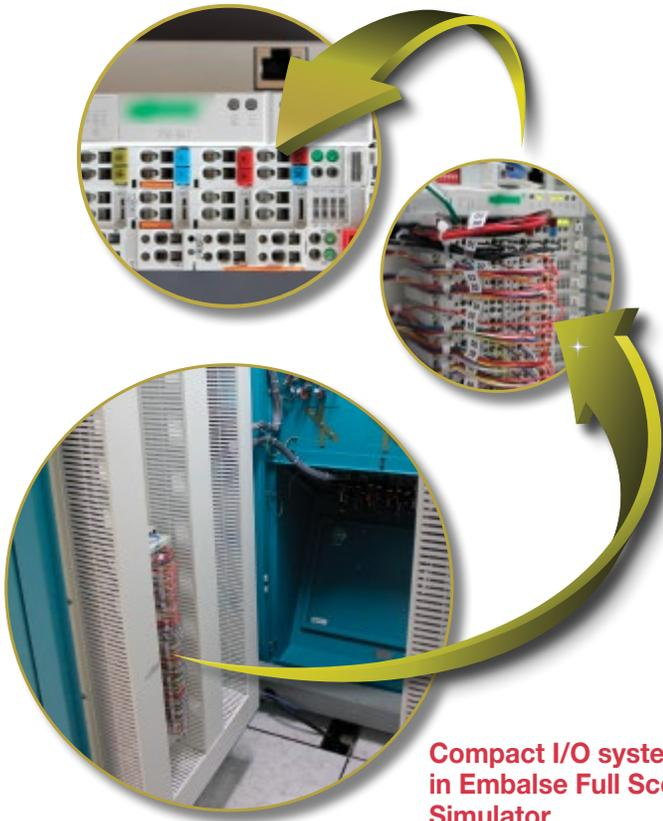
**Compact I/O system in Embalse Full Scope Simulator**
